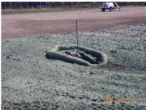
Straw Wattle Around Culvert
