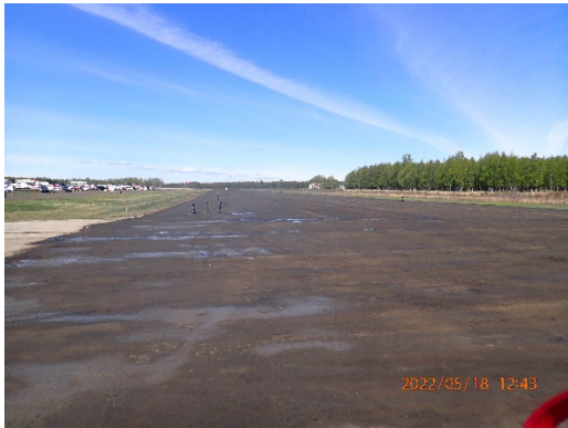
Finished Runway Rehabilitation Project
