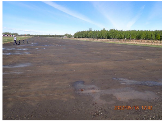
Finished Runway Rehabilitation Project
