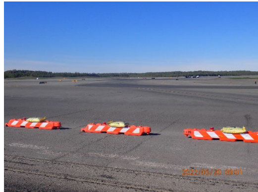
Next Phase of Runway Reconstruction
