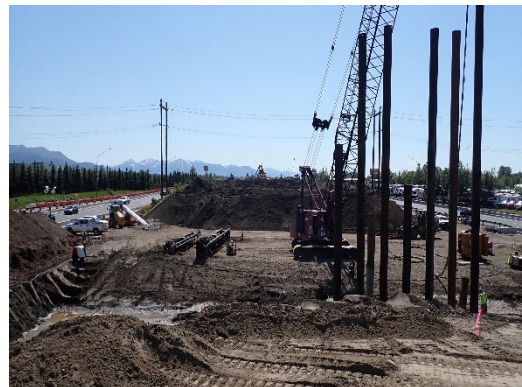
Overview of Seward Hwy bridge work
