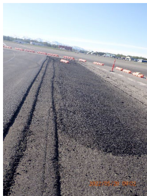
Current Phase of Runway Reconstruction
