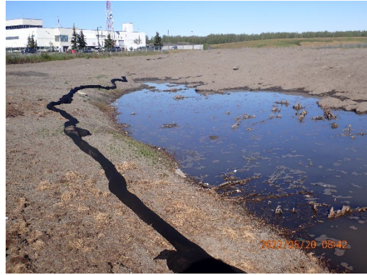
Comp Sock in Employee Parking
