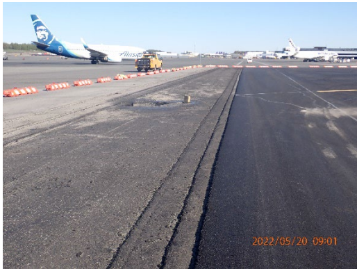
Current Phase of Runway Reconstruction
