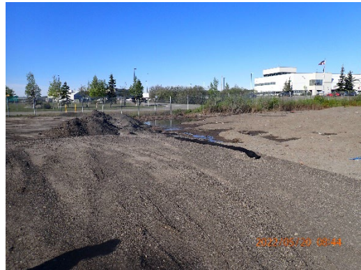
Comp Sock in Employee Parking
