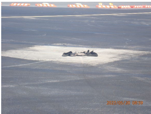
Witches Hat in Storm Water Grate
